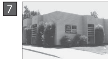
7 Turlock Medical Office 800 Delbon Avenue Suite A Turlock, CA 95382 664-8000
